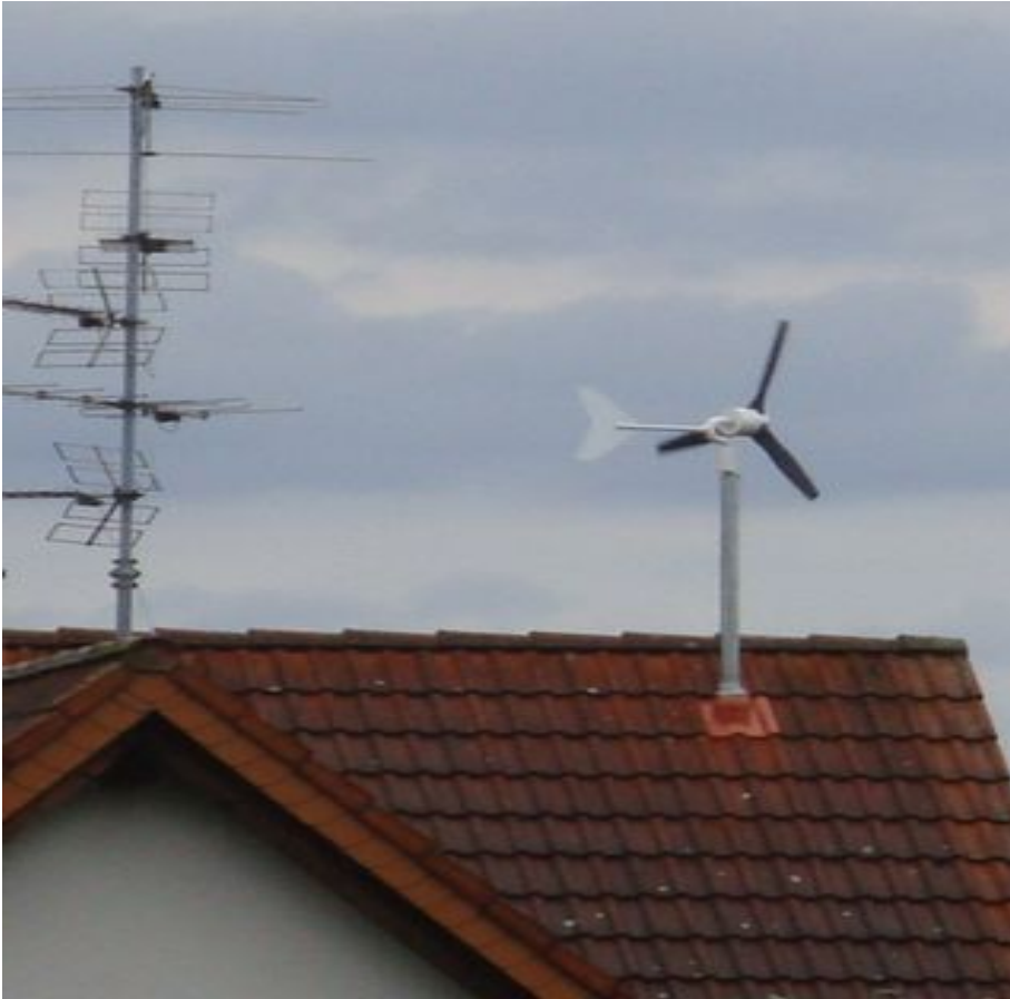
Figure 6 Example of a micro wind turbine used for a home. Source; https://energyeducation.ca/encyclopedia/Micro-wind_turbine
